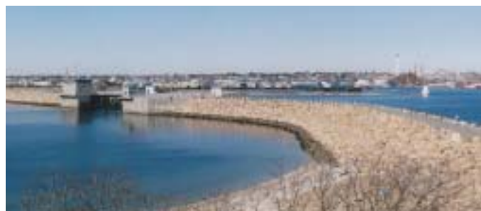
NEW BEDFORD-FAIRHAVEN-ACUSHNET HURRICANE BARRIER
