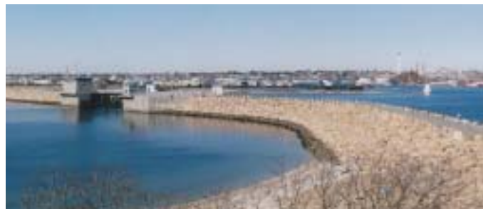
NEW BEDFORD-FAIRHAVEN-ACUSHNET HURRICANE BARRIER
