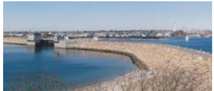
NEW BEDFORD-FAIRHAVEN-ACUSHNET HURRICANE BARRIER
